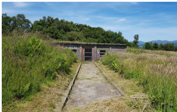
After Groundwork and Grills Fitted
